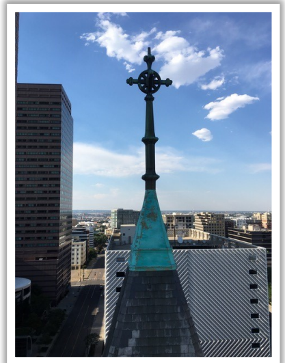
Steeple after repair
